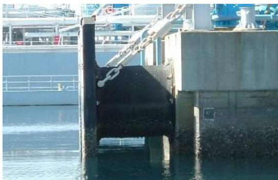
Fig.1 - Photo of Circular Shaped Buckling fender
